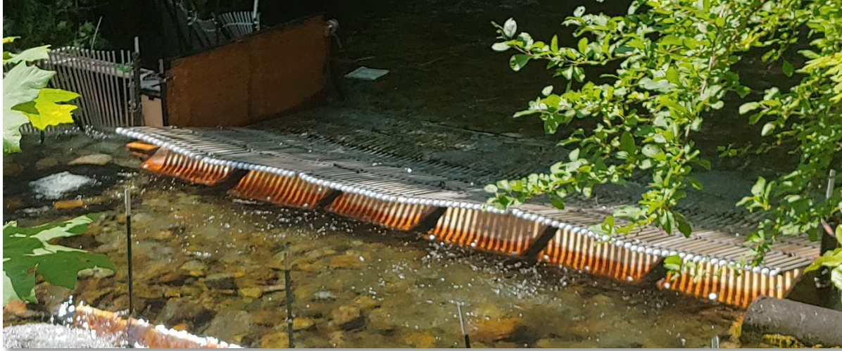
Figure 3. Photo depicting the aluminum picket leads, resistance board weir panels, video chute and camera chamber deployed in Cougar Creek.
