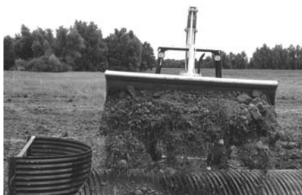
Lofton water control structure USFWS Photo
