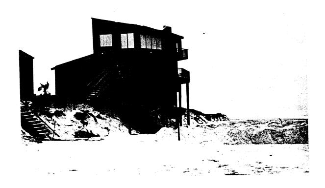
Figure 3-6. Undermining by Hurricane Allen of one of the units at the "Lost Colony" condominiums at Mustang Island, Texas. This illustrates that dune-scrap retreat is the typical storm response on a high-profile barrier island. Picture taken on August 15, 1980, five days after landfall of Allen. Mounds of sand on the right have been dumped there by truck after the storm. Contrast this with the storm-response of a low-profile barrier as seen in Figure 2-6.
