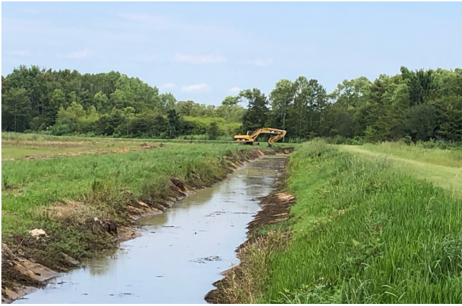
Ditch cleaning in managed impoundment by USFWS
