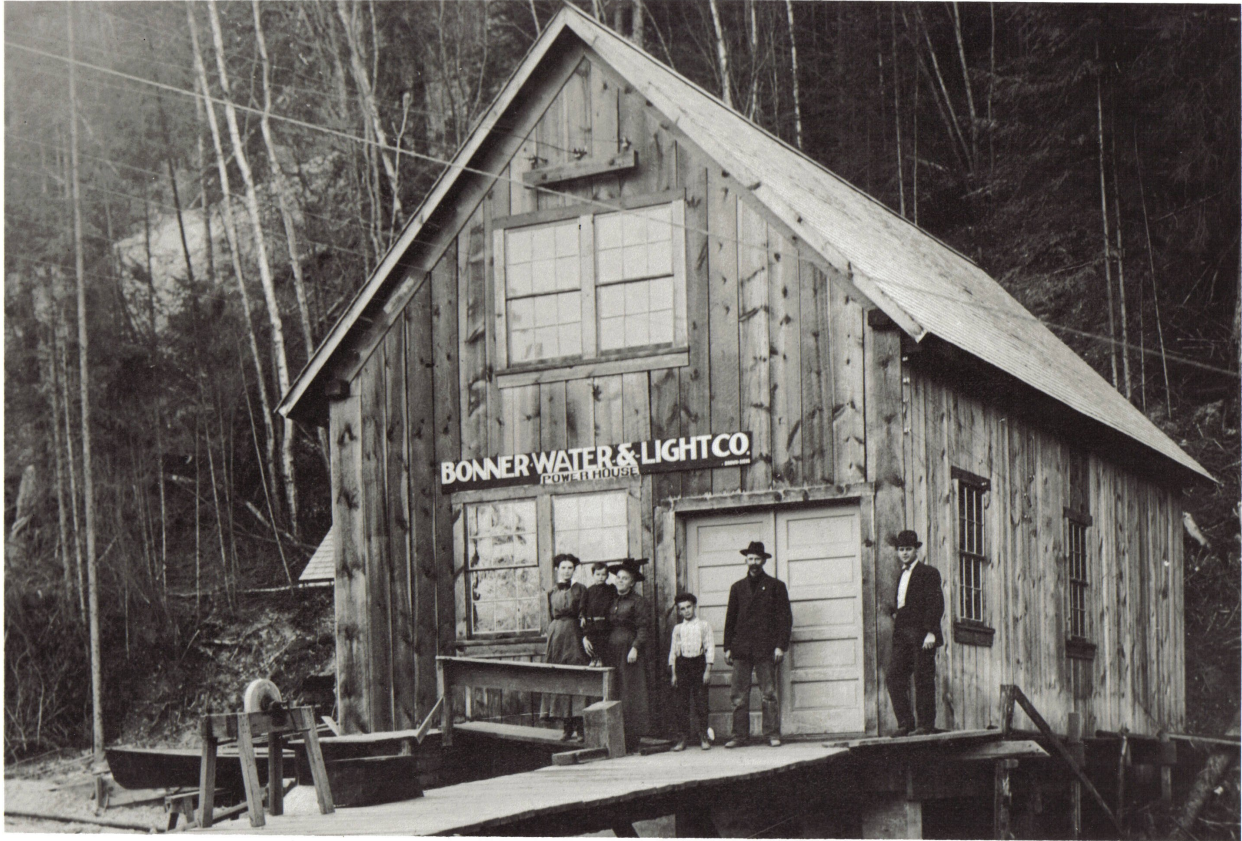
Figure 6.4. Bonner Water and Light Company powerhouse on Myrtle Creek, circa 1906. Photo courtesy Boundary County Historical Society.
