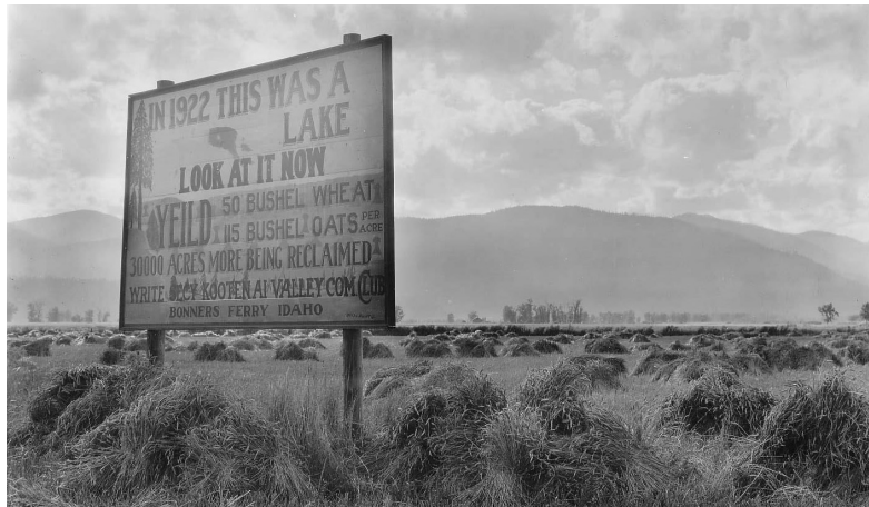
Figure 6.5. Sign on Diking District # 1, circa 1940. (USACE Seattle District Archives).
