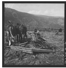
Figure 6.9. Ex-mill worker clears 8-acre field after bulldozer has pulled the stumps. Boundary County, Idaho.
