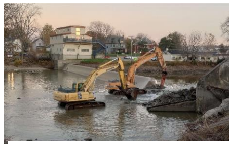
Charles Mill Dam Construction project; Photo credit: Jerry Sweeten EcoSystems
