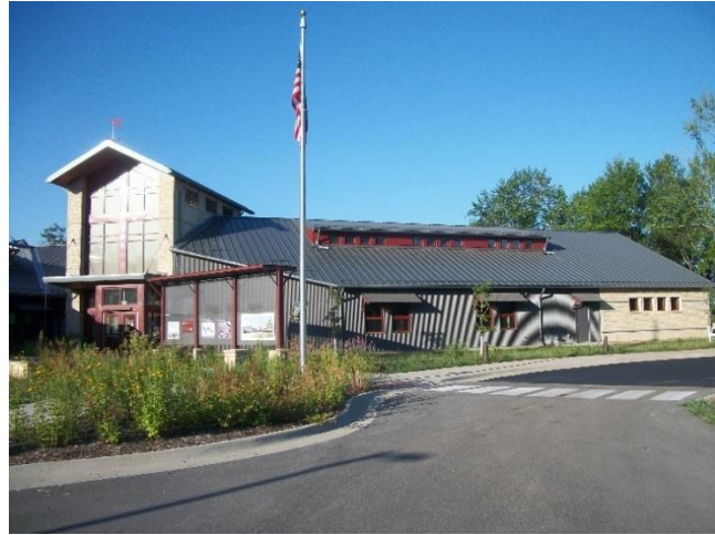
Crab Orchard NWR – Replacement Visitor Center, completed in August 2023. Credit: USFWS
