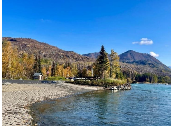
Kenai NWR – Replacement Boat Launch, Parking Improvements and Public Restrooms at Jim’s Landing. Credit: PND Engineers, Inc
