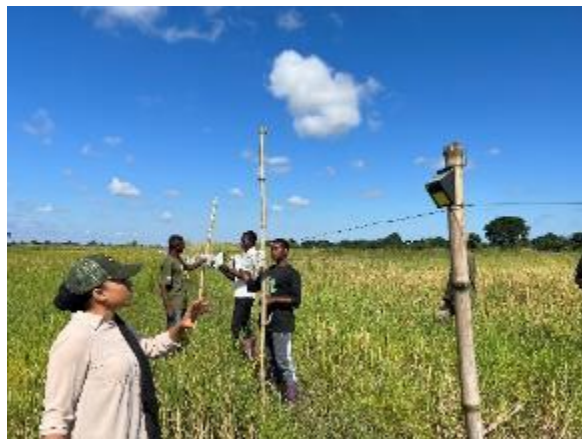
By adding metal strips and strobe lights to fencing, elephant crop raiding dropped by more than 50 percent. Credit: Matthew Luizza/USFWS
