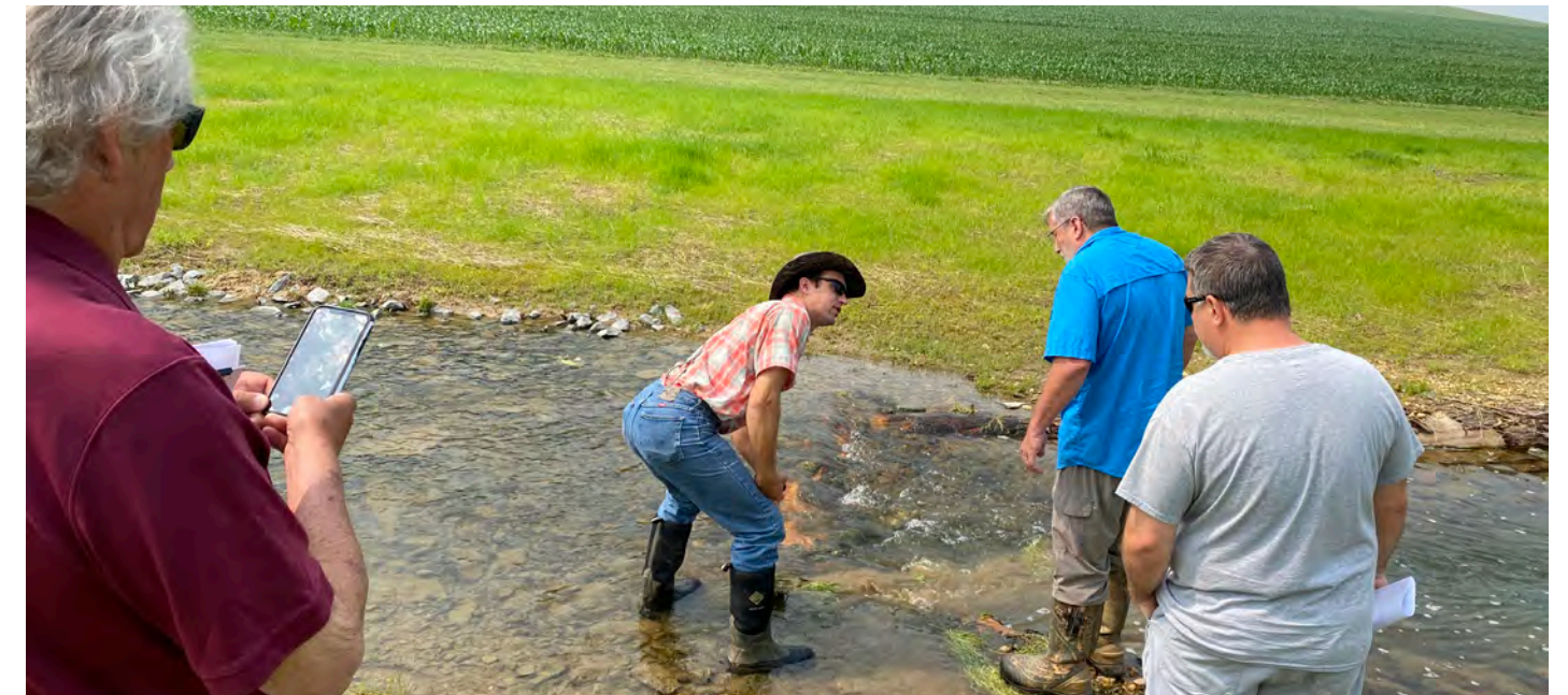
USFWS, Unique Excavating and Pheasants Forever staff, working to restore Indian Spring Run and an adjacent cold-water tributary. ©USFWS.
