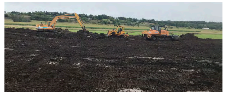
Heavy equipment excavating a depressional wetland. ©USFWS.
