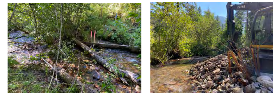
A view of the unscreened irrigation ditch, looking downstream (left), The formerly unscreened ditch was plugged with on-site sediments, backed by geotextile fabric, and reinforced with willow transplants (right). ©USFWS.
