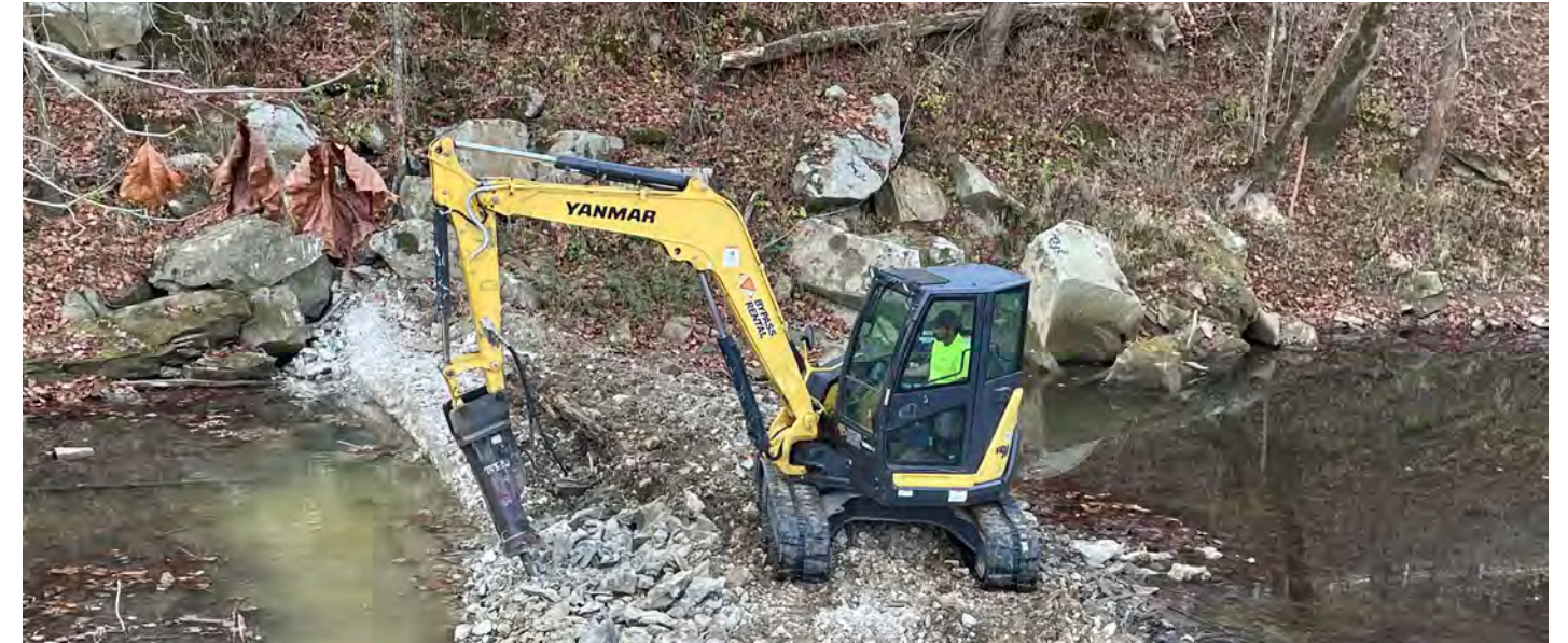
Heavy equipment notching the dam as part of barrier removal. ©USFWS.
