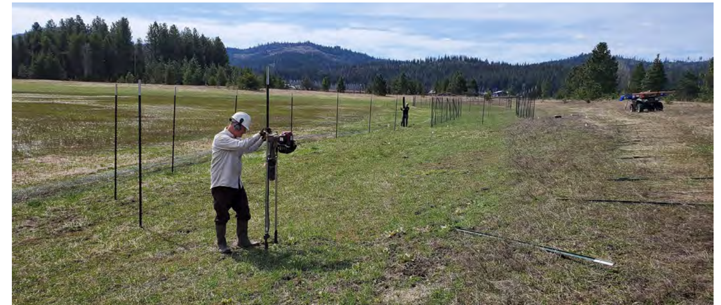
Installing 10 foot t-posts and 7 foot tall deer fencing to keep deer, elk, and moose from uprooting newly planted trees and shrubs. Photo credit: Ducks Unlimited.
