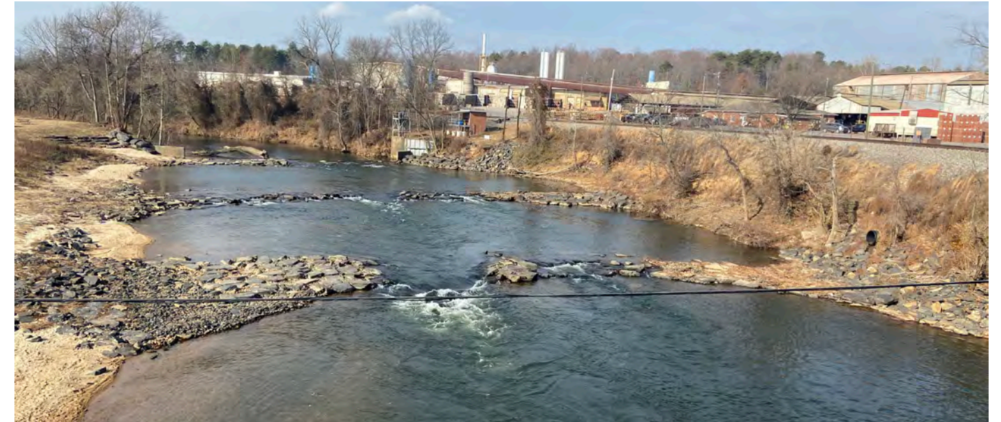
A series of weirs replaced the Lindsey Bridge Dam opening up 48 miles of previously inaccessible stream reach. Credit: K. Bass
