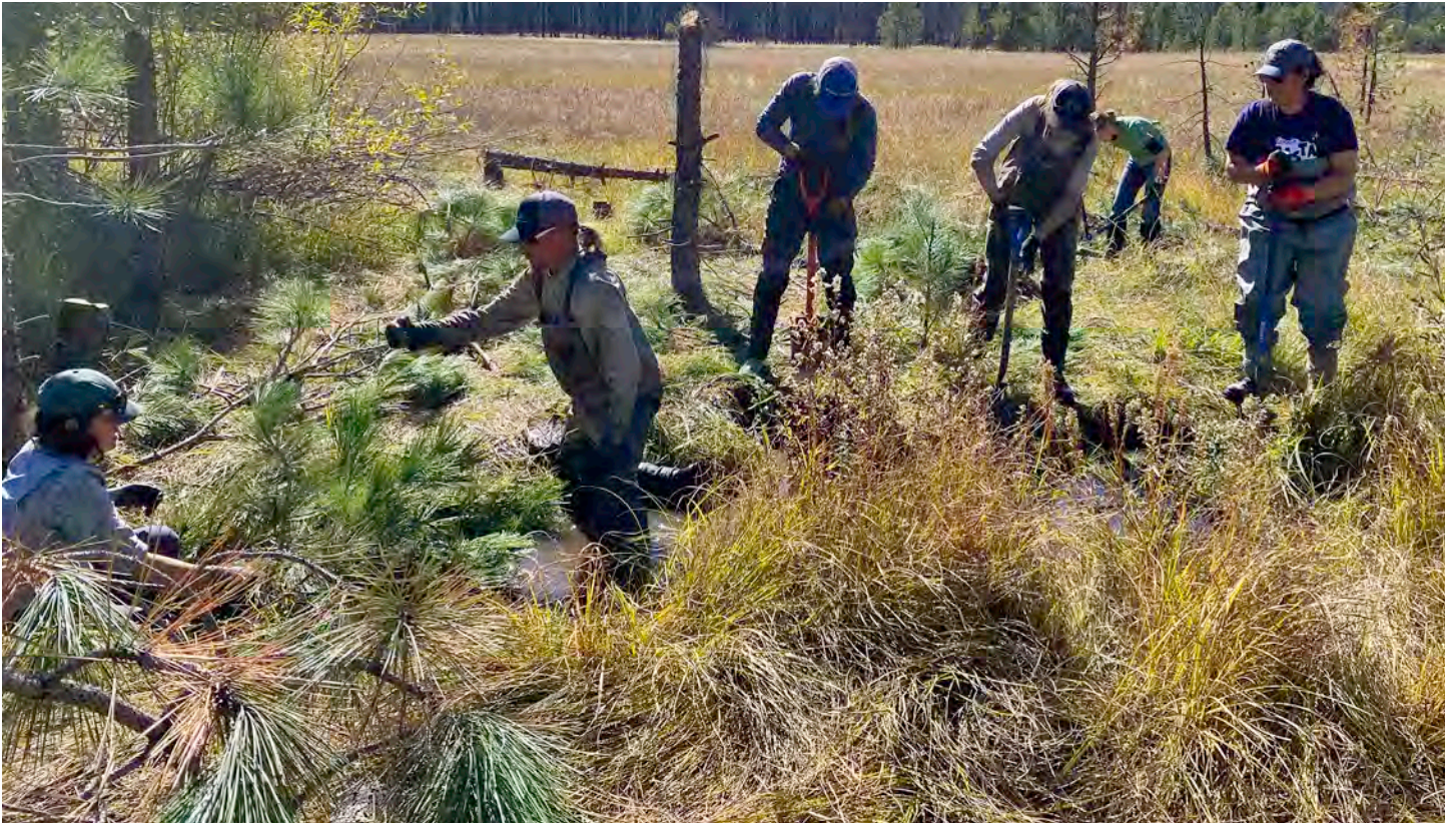
Above: Process-based restoration workshop attendees building structures (California). ©USFWS.
