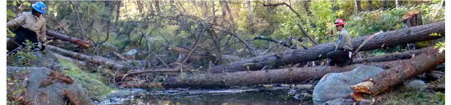
PFW is a leader within the Department of Interior in implementing Nature-Based Solutions by delivering conservation projects such as stream restoration, culvert replacement, fish passage, fuel management, pollinator gardens and reforestation. Photos ©USFWS.
