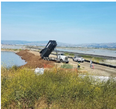
Soil delivered to Pond A12 for levee construction.
