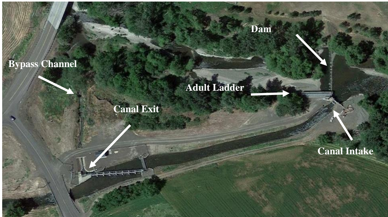
Figure 19. Aerial photo of Burlingame Dam (rkm 61) on the Walla Walla River near Milton-Freewater, Oregon. The diversion dam, canal intake, canal exit, fish bypass channel and adult fish ladder are indicated. (Photo derived from Google Earth Pro, Imagery Date: 6/13/2019).
