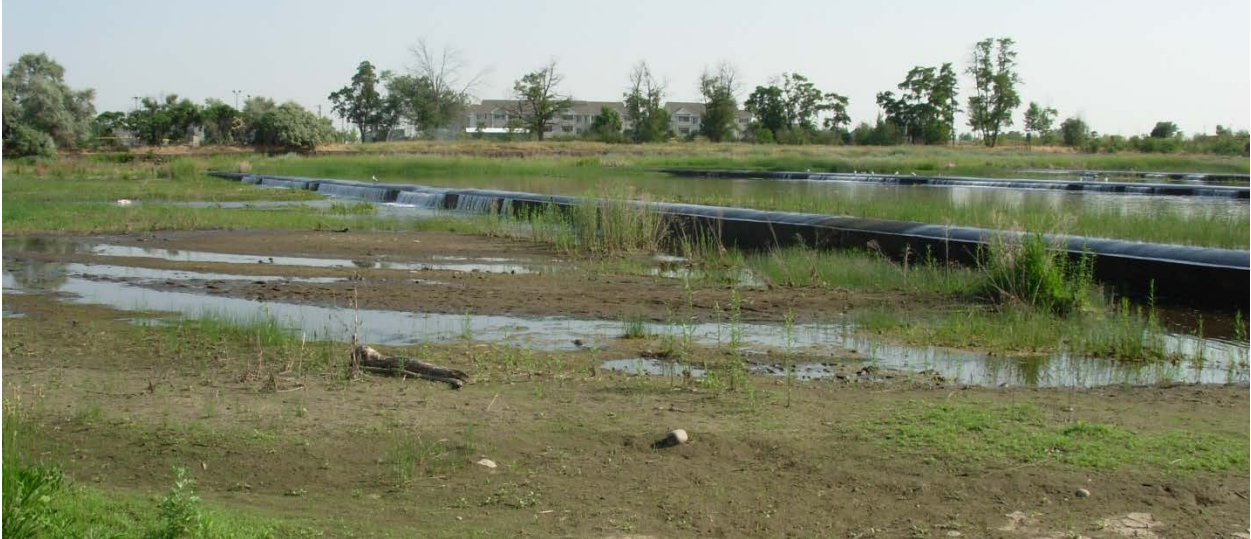
Figure 3.69. Example of stabilization sills near the downstream bound of reach MC18 (approximately rkm 15) as surface flows decline during early summer months in Mill Creek near Walla Walla, WA.
