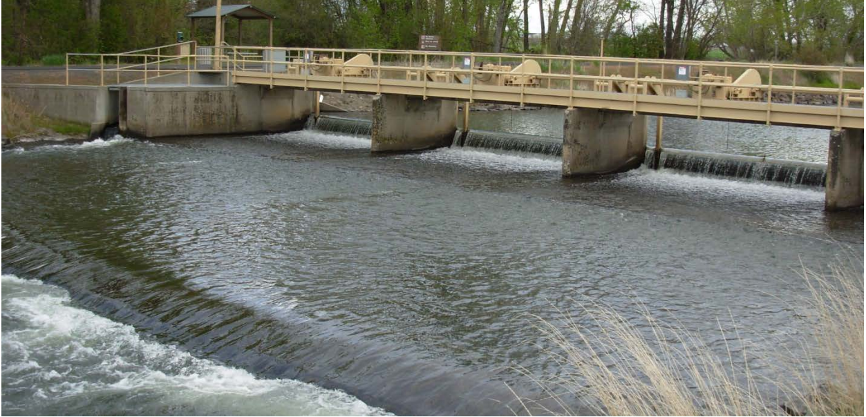
Figure 3.59. Mill Creek Division Dam on Mill Creek near Walla Walla, WA.
