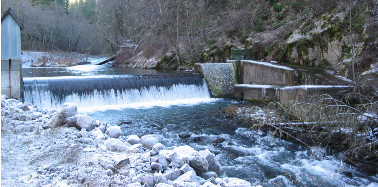
Figure 3.45. The City of Walla Walla Intake Dam and associated fish ladder at the downstream boundary of reach MC14 (rkm 44.2).
