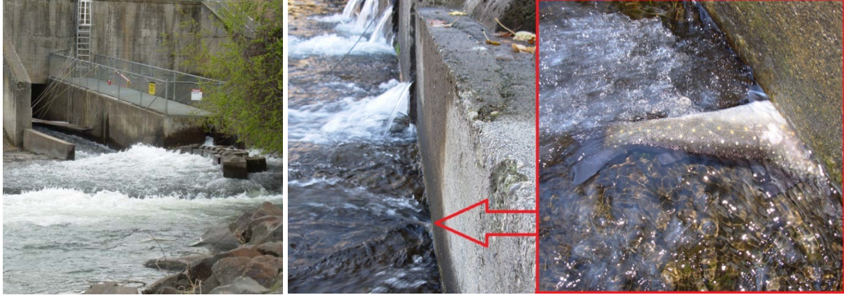
Figure 3.63. Low flow outlet and fish ladder entrance (left), eco-block separation wall (center) and impinged adult-sized bull trout (right) at the Mill Creek Diversion Dam in Mill Creek near Walla Walla, WA.
