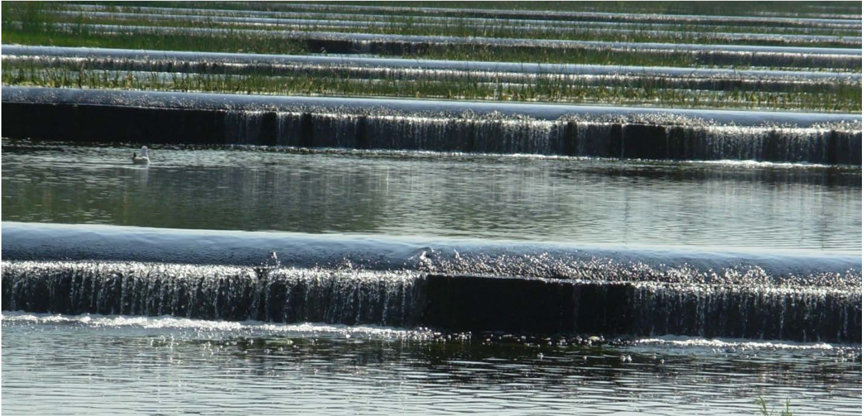
Figure 3.60. Gabien-style concrete sills downstream of the Mill Creek Division Dam on Mill Creek near Walla Walla, WA.
