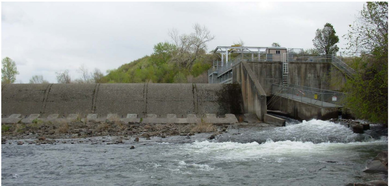
Figure 3.62. Mill Creek Diversion Dam on Mill Creek near Walla Walla, WA.
