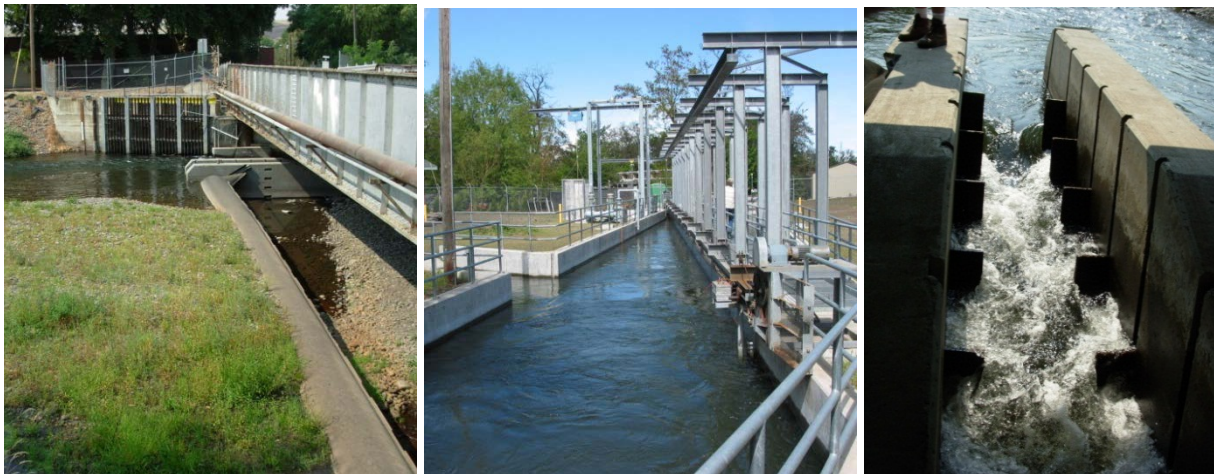
Figure 3.54. Photographs depicting the inflatable dam (left), diversion canal (center) and fish ladder (right) at the Little Walla Walla Diversion facility (rkm 75.1) on the Walla Walla River near Milton-Freewater, OR.
