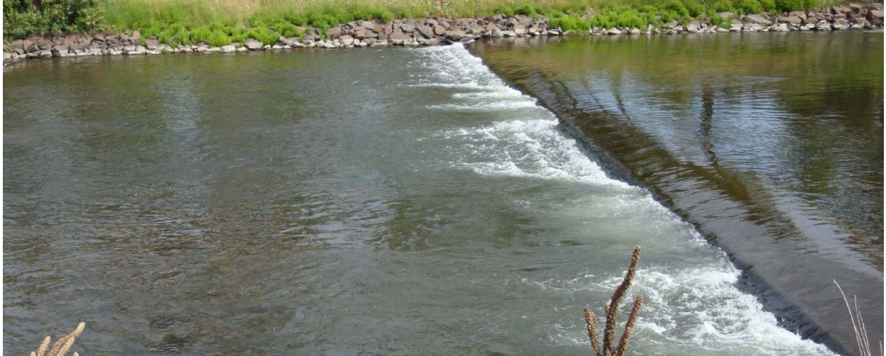
Figure 3.67. Scoured pools immediately downstream of stabilization sills within the flood control project in reach MC17 (approximately rkm 19) near Walla Walla, WA.
