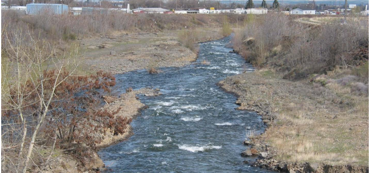
Figure 3.53. Levee section downstream of Nursery Bridge Dam (reach WW7) on the Walla Walla River near Milton-Freewater, OR.
