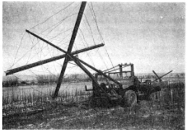
*Fig. 4: Jack unit is moved to position in jetty field by a winch controlled lift. Casa Colorado area, Middle Rio Grande Project, NM. Photo:Herman E. Carter, Bureau of Reclamation (Carlson and Enger 1956).*
