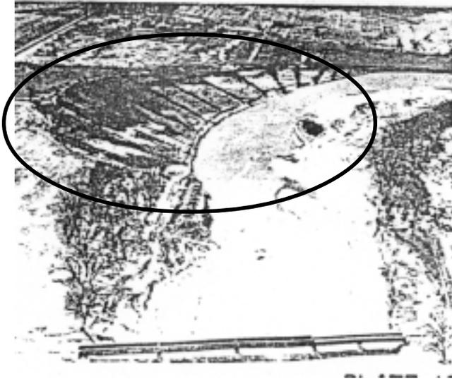
*Fig. 7: A jetty field was installed in 1947 by the A.T. & S.F. Railway Co. The photo left is from 1949 and shows the results of the jetty project. The system used a total of 980 jack units: 40 feet of retards, 1800 feet of double diversion lines, and 14 backup retard lines. The jetty field is still visible on the upper bank of the river (U.S. Army Corps of Engineers 1953).*
