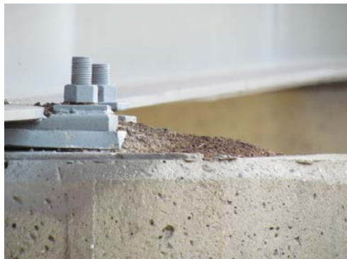
Photo 5: Guano deposit on pier, obscuring structural features.
