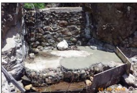
McKnight barrier with newly laid concrete.
