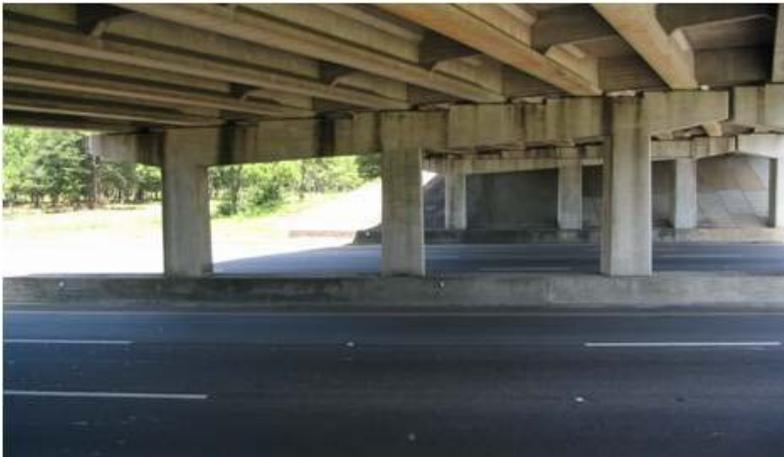
Photo 9: Staining on sides of pier caps
