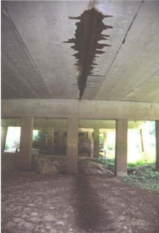
Photo 7: Staining along longitudinal joint.
