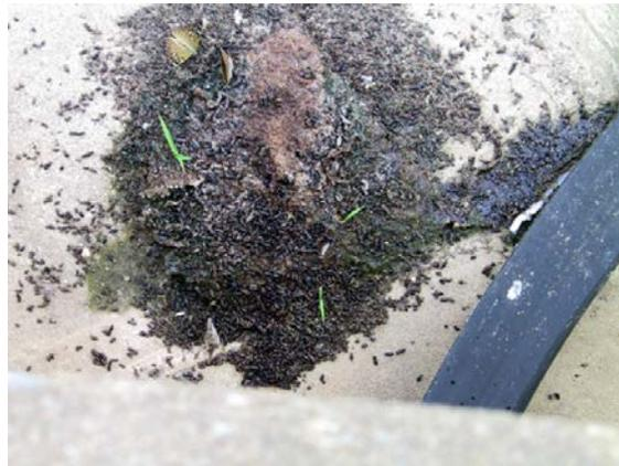
Photo 4: Guano deposits visible from bridge deck, on top of pier
