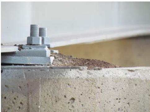
Photo 5: Guano deposit on pier, obscuring structural features.
