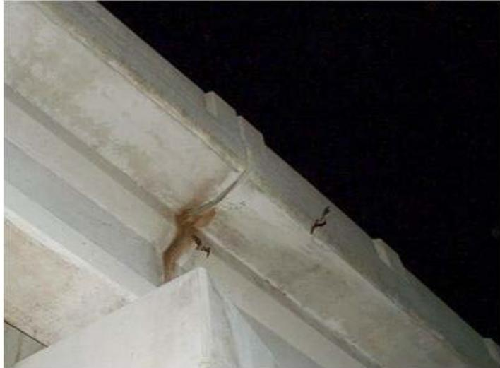
Photo 8: Staining on underside of expansion joint from bat use.
