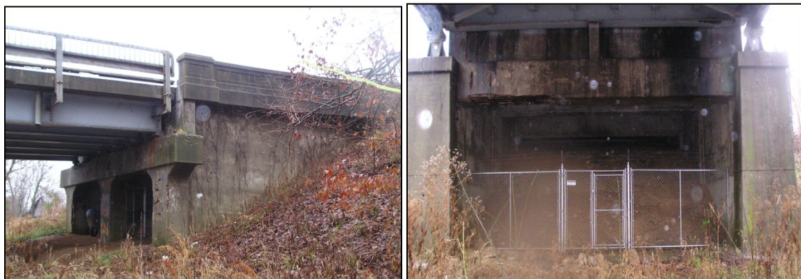
Photo 12 and 13: Bridge design mimicking “cave-like” atmosphere
