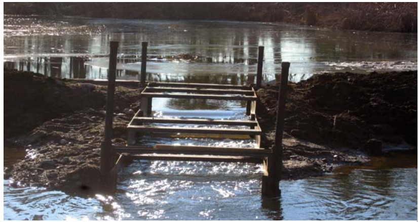
Fish ladder to pass northern pike and muskellunge to spawning and rearing habitats, Delaney Bay, St. Lawrence River, Grindstone Island, New York. Ducks Unlimited, U.S. Fish & Wildlife Service Partners for Fish and Wildlife, and SUNY-ESF.
