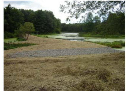
Spillway and drain restored
