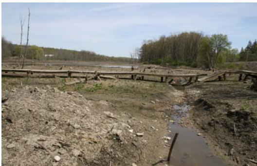
Damaged by beaver activity and Susquehanna River flooding
