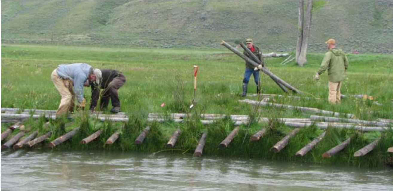
Above: Workers assemble logs around newly-planted willows, securing the logs in place to reduce movement. Below: A clump of willows near Flat Creek shows the effects of heavy browsing.
