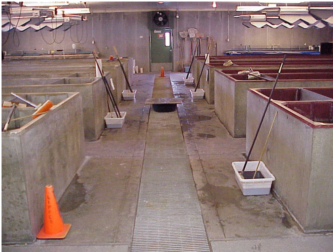
Figure 1. Tank room at Murray Springs Trout Hatchery.
